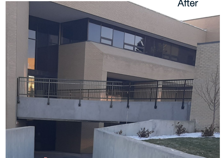
Mazurek Bridge Replacement, DOA
