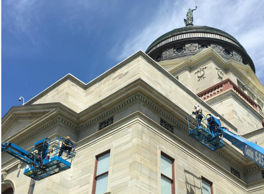
Comprehensive Condition Assessment MONTANA STATE CAPITOL
